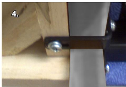
Step 4: Place the chairs that will be attached to the connecting table approximately 24" apart. Carefully place the connecting table top facing up on the 4 suspended "L" brackets. Using the 4 bolts and washers removed in Step 1, attach the table to the chairs. Do not tighten the bolts until the chairs are in their final location. Be certain that the table is snug against the chair frame.
